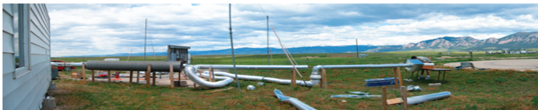
Figure 5. Dynamic characteristics and an actual photo of the flare facility design.
